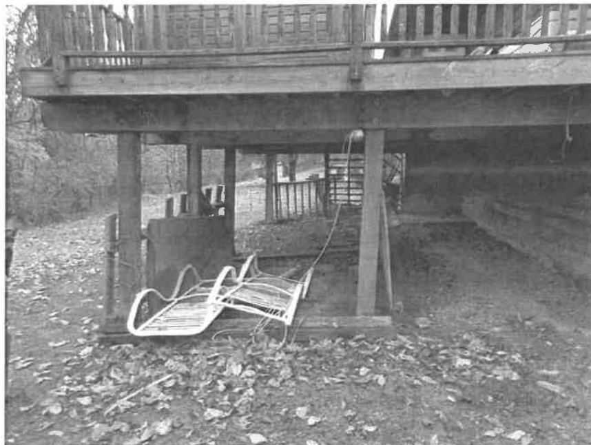
Photo No. 3: Improperly supported deck posts and hot tub. The posts are supported on masonry blocks laid on the ground surface without a foundation.
