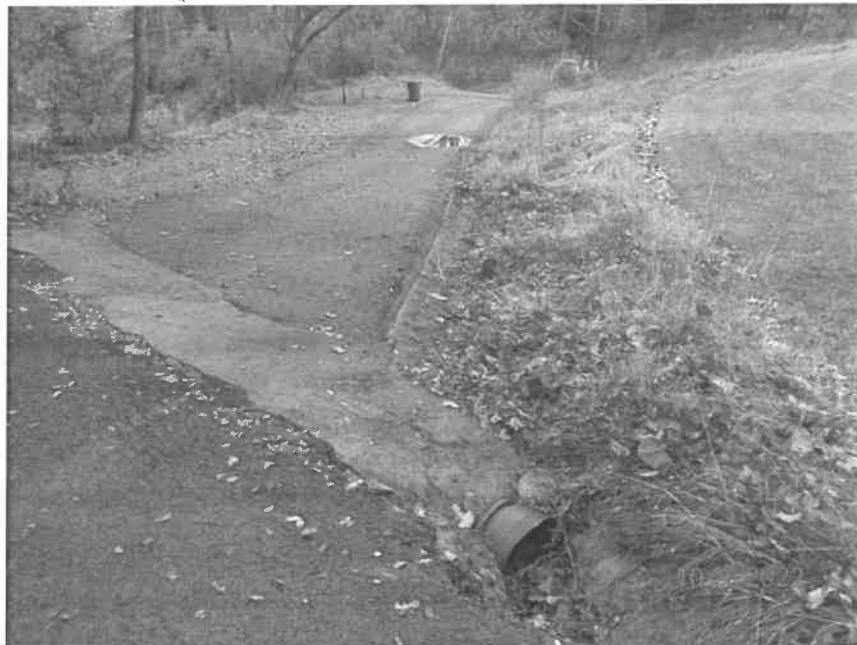
Photo No. 10: Slide scarp and repair with new drain pipe.
