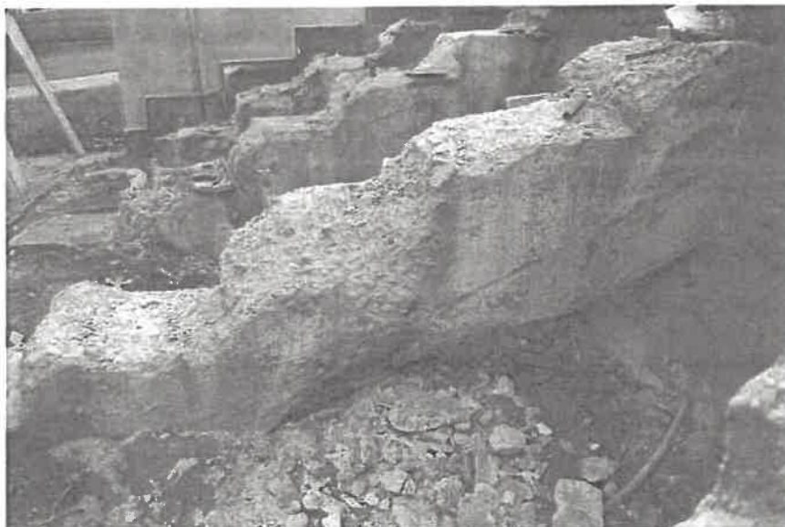
Photograph 3. Example of deteriorated concrete stringers beneath side stair
