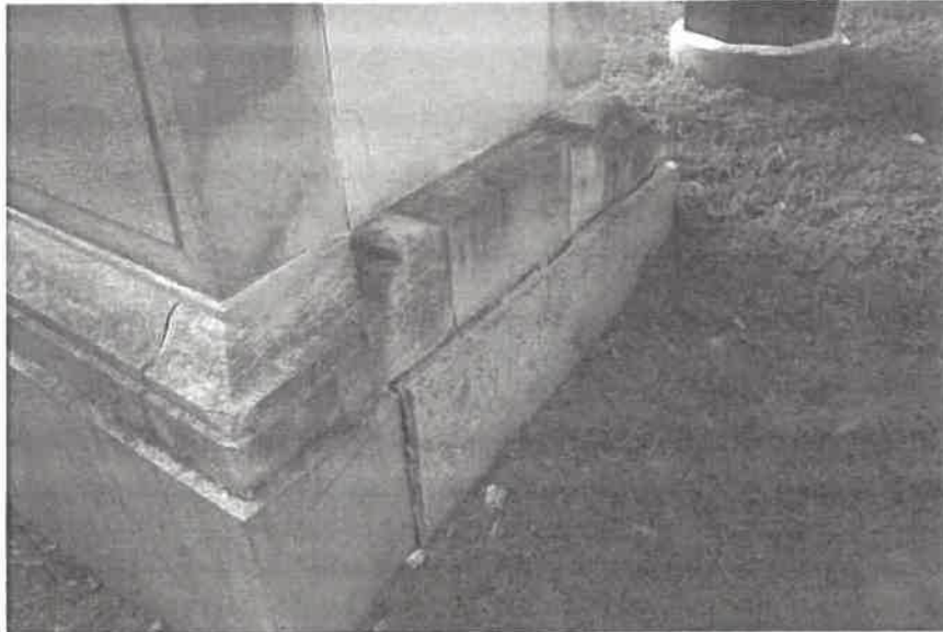
Photograph 2. Example of separated granite panel at side pillar
