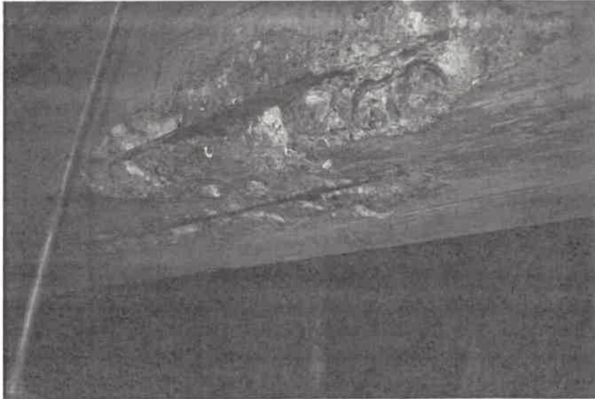
Photograph 4. Example of concrete and reinforcement deterioration and concrete beam beneath platform
