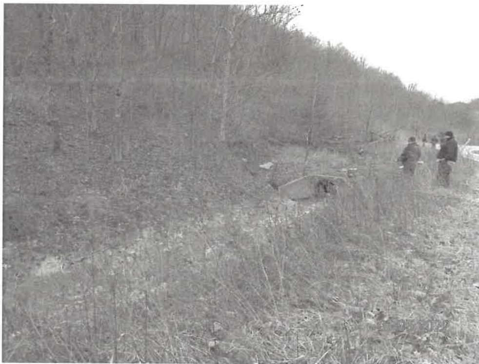
Photo No. 14: RCP inlet facing north and erosion/overflow area just north of the inlet.
