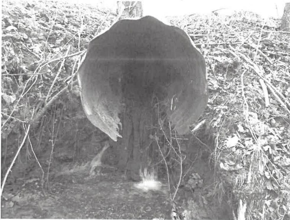
Photo No. 2: Impoundment drain pipe outlet. Blocked on the upstream end and consumed by corrosion.
