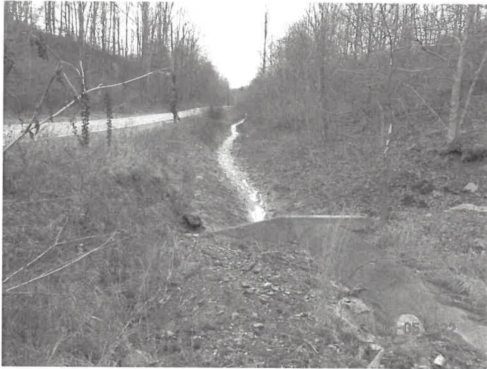
Photo No. 13: Existing grouted rip rap channel carrying Fords Run to the 48" RCP.
