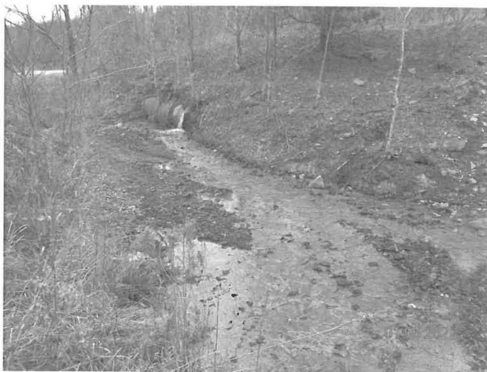
Photo No. 12: AMD and leaking 48" RCP carrying Fords Run.
