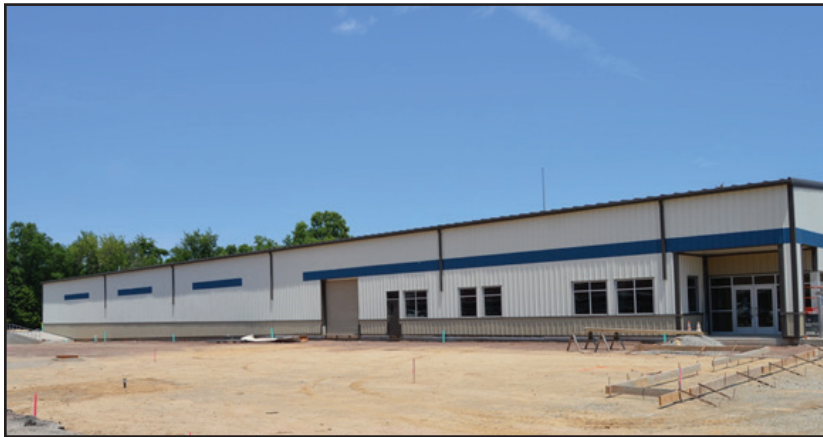
Progress continued during Fiscal Year 2016 on the new office and warehouse structure at the West Virginia State Agency for Surplus Property in Dunbar, West Virginia. The new building replaced the previous facility that was built in the 1950s.
