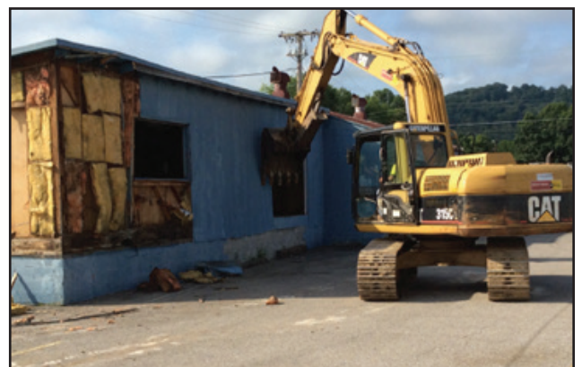
The first building to be demolished was the former "auction room," which was previously used by the state carpenter in the 1980s.
