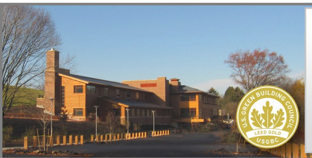
Harvard University Arnold Arboretum Weld Hill Research and Administration Building
