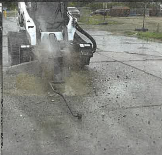
PUSH SPOIL MATERIAL TO THE SIDE SO YOU WON'T COMPACT IT
