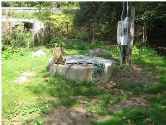
Before: Upper Drive Lift Station
