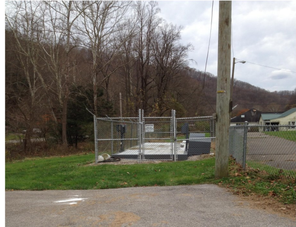
Existing Package WWTP to be Abandoned
