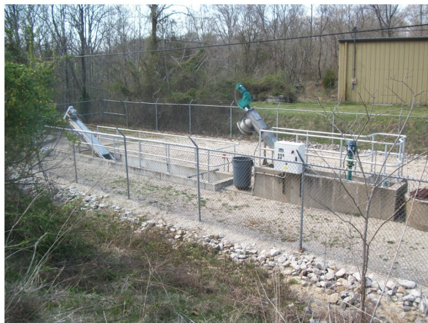
Terminus of Project at Existing Ona West Pretreatment Facilities
