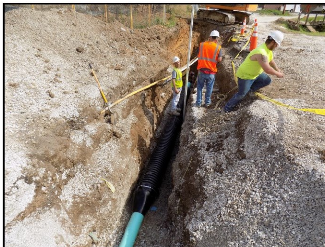
Sanitary Sewer Line Encasement at Water Line Crossing
