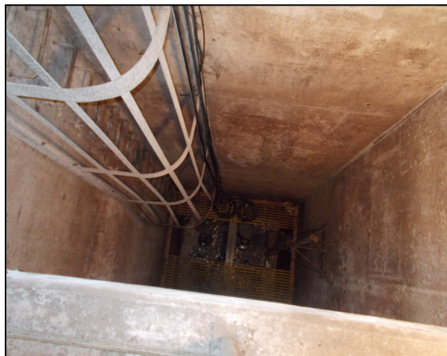
Wet Well of Pump Station to be Rehabilitated
