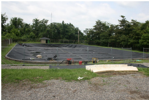
Reservoir Floating Cover Replacement
