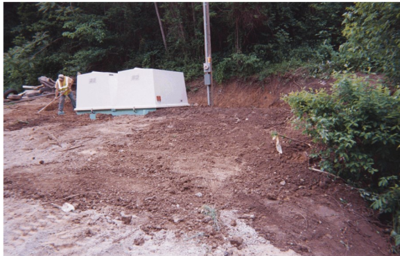
New booster station during construction.
