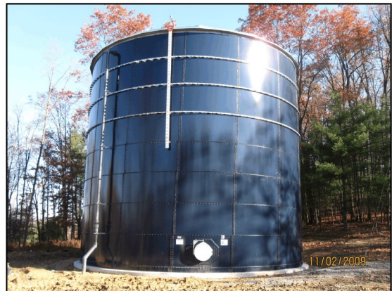
402,000-Gallon Water Storage Tank
