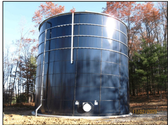
402,000-Gallon Water Storage Tank
