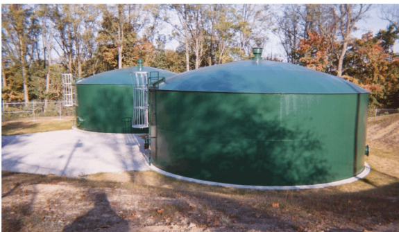
Two new water storage tanks.
