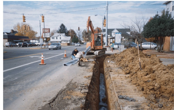
Replacement of water line along US Route 60.
