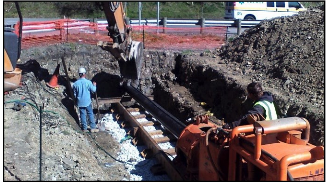
Bore and Jack Crossing of Corridor G/US 119
