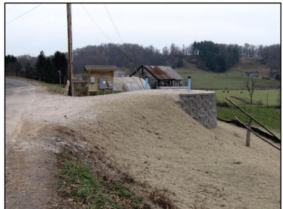
50 GPM Booster Station
