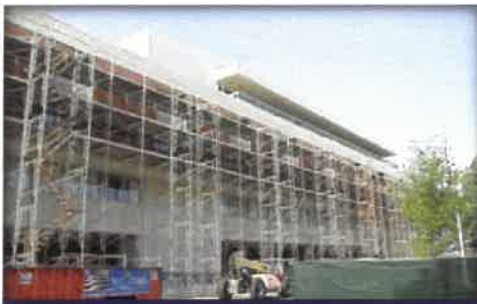
Temporary protection for façade replacement project of occupied building.
