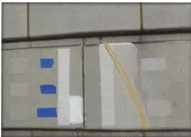
Masonry Repair Material Trial Installation for Historic Preservation
