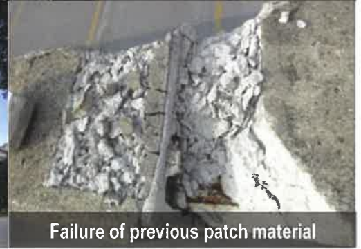
Full-depth Slab Repair
