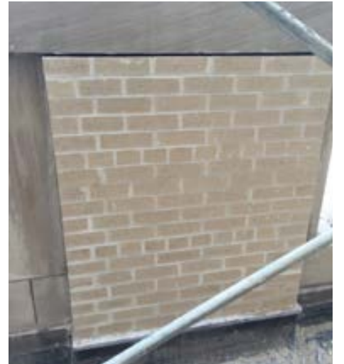
Reconstructed parapet mitigates water infiltration
