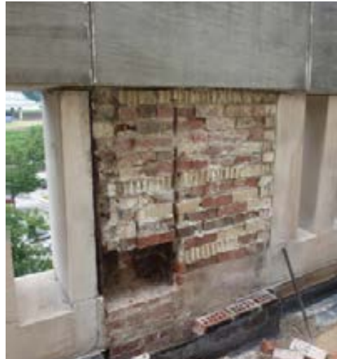
Parapet during exploratory demolition
