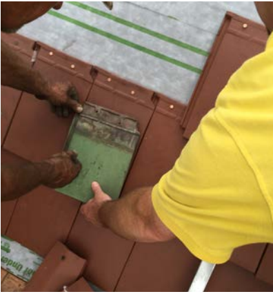
Mockup of new roof as part of QC
