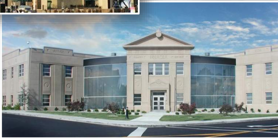
Mercer County Courthouse Annex
