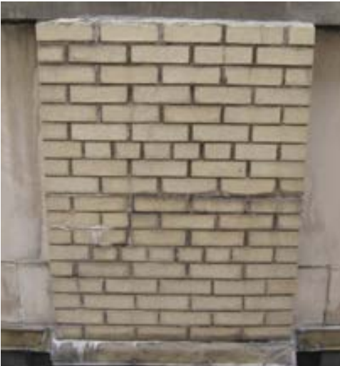
Parapet existing condition
