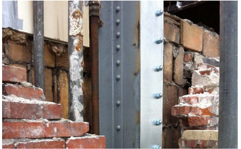
Forensic field investigations revealed significant deterioration of masonry and steel at the terra cotta frieze, balustrade, and lintels above the windows.
