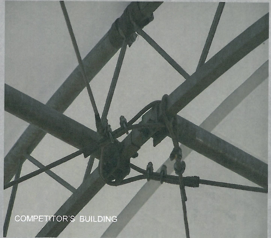
CABLES WRAPPED AROUND SADDLE BRACKETED PURLINS
