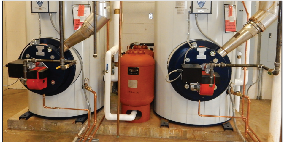
The Division of Corrections has awarded several open-end maintenance contracts. These contracts, such as the contract that provides service for two 400-gallon domestic hot water heaters at Anthony Correctional Center, allow the Division to respond quickly to equipment malfunctions.
