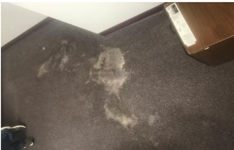
Visible Mold Growth & Water Staining on First Level Carpet
