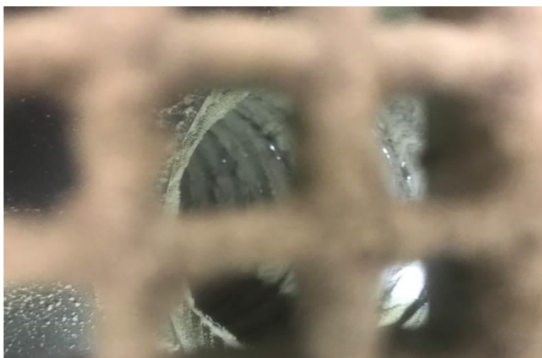
Visible Dust Accumulation on HVAC Ductwork
