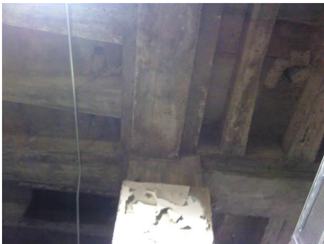
First Level Microbial Growth on Column show current water infiltration
