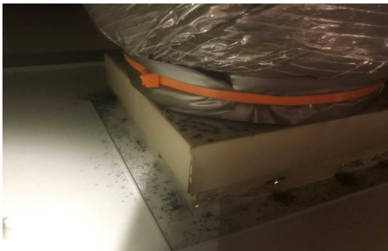
Visible Mold Growth on Supply Diffuser
