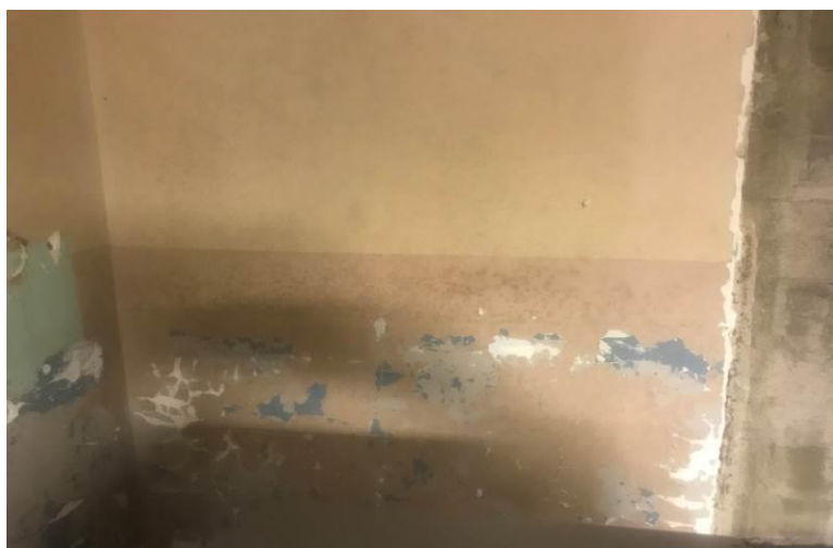
Visible Mold Growth on Plaster Walls
