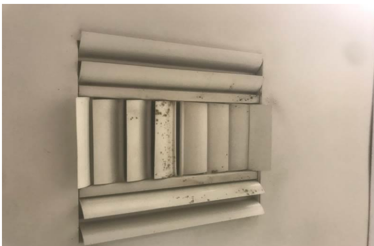
Visible Mold Growth on Supply Diffuser
