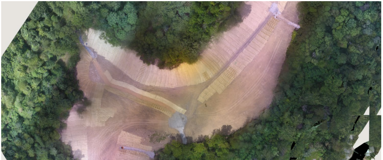
Canyon Run AML – As-Built Monitoring – 2020
