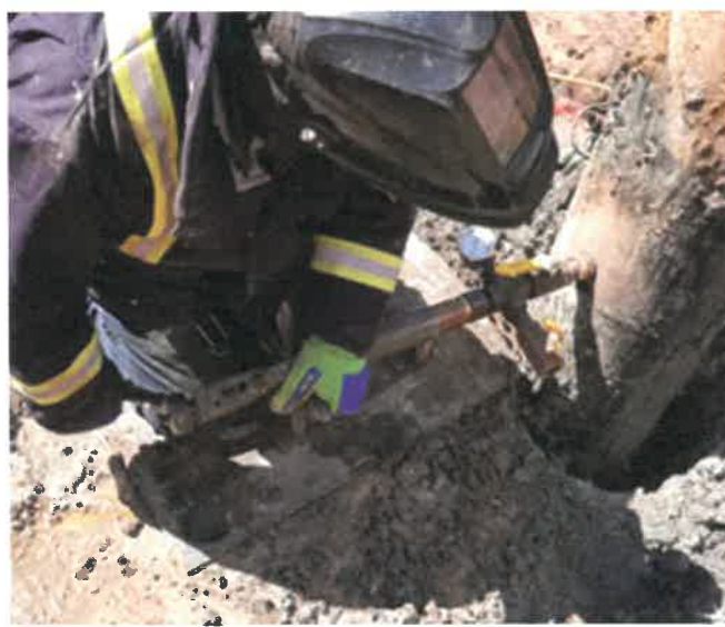
FIGURE 2-5: COLD-TAPPING OPERATIONS
