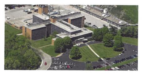
Typical modern laboratories maintain humidity control which means humidification during the heating season. As the building exists, condensation will occur on the interior face of the window and curtain wall system. If humidity control is desired, replacement of the curtain wall is necessary.
