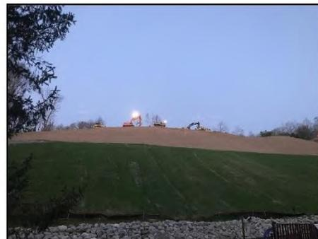
The final design of the stabilized hillside resulted in three benches and well over 100,000 cubic yards of material excavated and placed. Due to the nature of onsite soils, POTESTA also utilized cement reinforced soils to allow for construction to advance even during the winter months.
