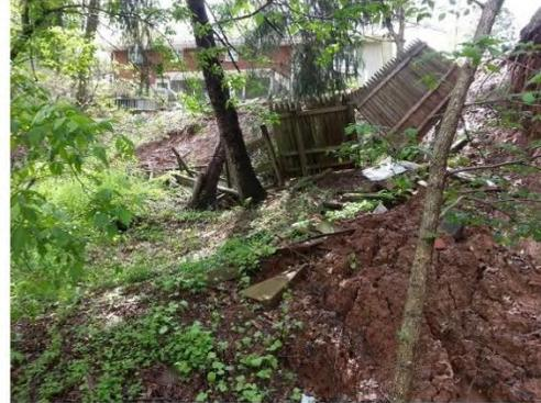
The work required the removal of all failed material to the underlying bedrock surface and included the installation of a shot rock toe buttress which was installed along a natural topographic bench near the toe. Following the completion of the slope repair, the affected utilities were installed either below or outside the limits of the regraded slide area.
