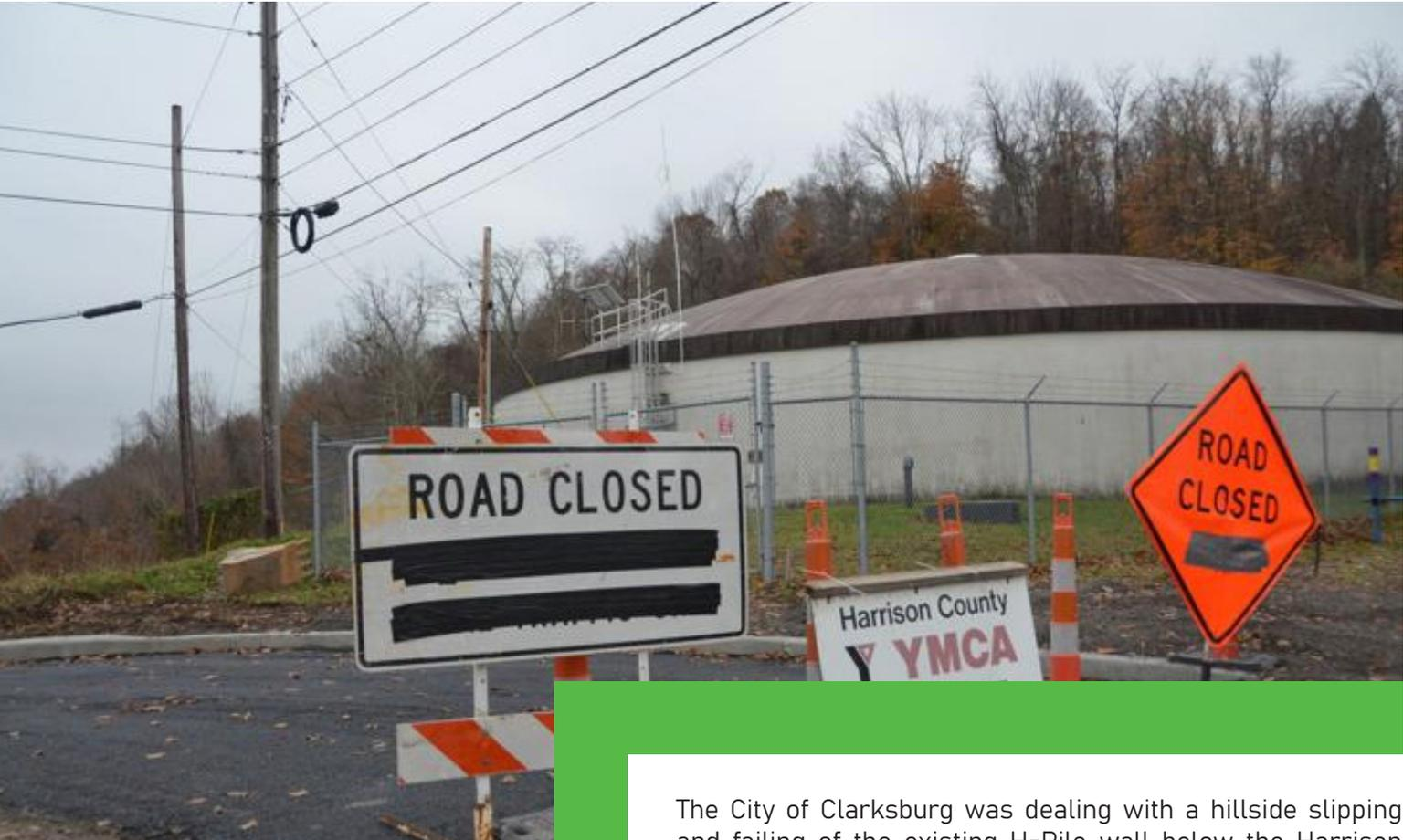
The City of Clarksburg was dealing with a hillside slipping and failing of the existing H-Pile wall below the Harrison County YMCA / Lowndes Hill Park and above Second Street. The Ascent team evaluated the area and slip cause to provide a plan for fixing the slip.
