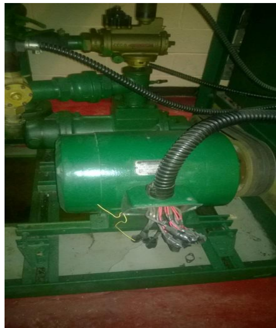
Make-shift Wiring Repairs
