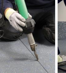
For corner weld, use a CA72 welding rod.
