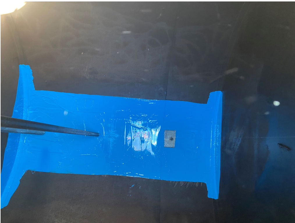
View of the gasoline compartment after application of epoxy coating by Superior Services
