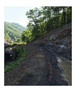
This project included `6,500 cubic yards of earthwork and stabilizing the slope behind the residence.
