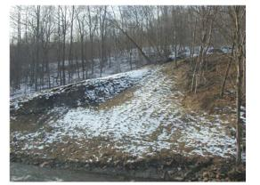
strata depths and water levels, using piezometers. Slope stability analyses were performed to determine the corrective actions required to stabilize the area. Surface and subsurface drainage structures, a toe key, and stream bank protection were designed to correct the instability problems and provide long term protection to the area.
