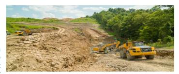
is to extend the existing runway by 1,001 feet, creating a safer takeoff and landing space for outgoing and incoming flights. Over 100,000 CY of rock excavation was part of the scope of the PH-1 project.
