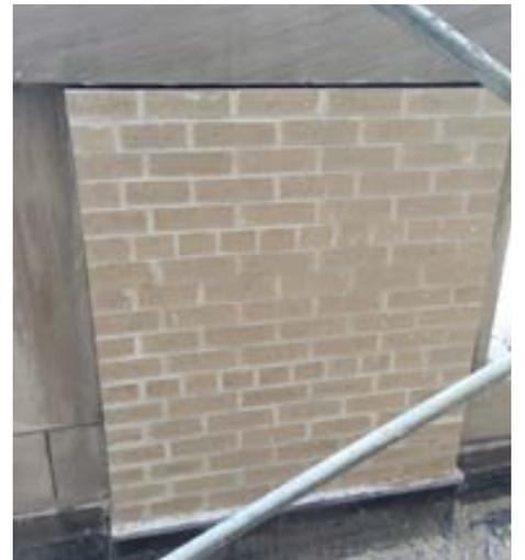
Reconstructed parapet mitigates water infiltration
