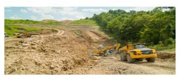
is to extend the existing runway by 1,001 feet, creating a safer takeoff and landing space for outgoing and incoming flights. Over 100,000 CY of rock excavation was part of the scope of the PH-1 project.
