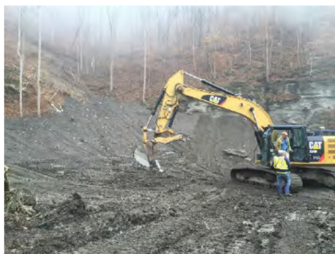
AML Highwall Grading
