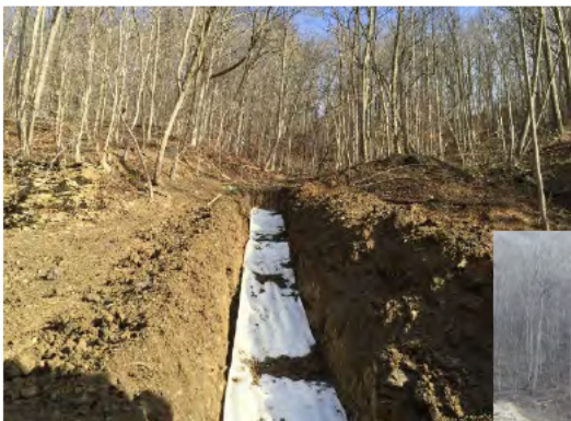
Liner Installation
