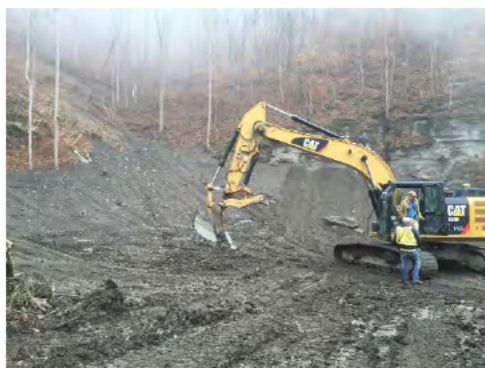
AML Highwall Grading
