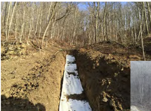
Liner Installation
