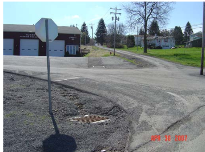
New Storm Drains and Catch Basins
