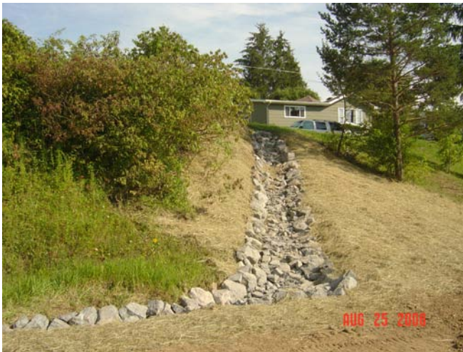
Erosion Repair – Rip Rap Armored Ditch
