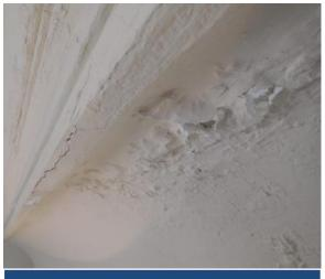
Moisture damage to run-in-place plaster
