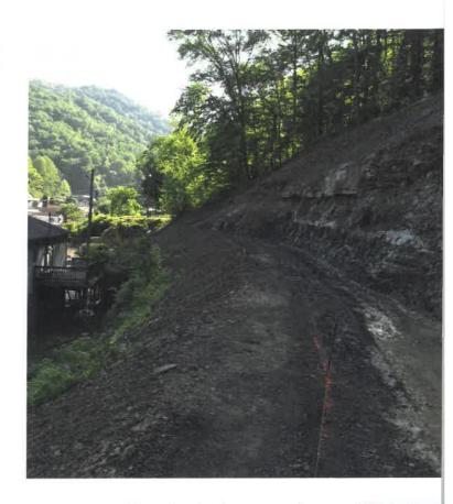
This project included `6,500 cubic yards of earthwork and stabilizing the slope behind the residence.
