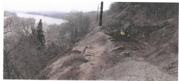
transmission line. Through field investigations and the design effort, a rock buttress was used to mitigate the landslide and avoid disruption to the power grid.
