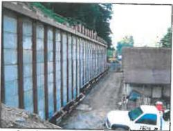
The retaining wall design required the application of a rock anchor tie-back system due to mine voids existing at the base of the hillside slope that were encountered during the subsurface exploration.
