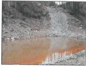
The Upper Muddy Creek project involved acid mine drainage from four areas that discharged into Muddy Creek upstream of where it crosses beneath State Route 3 (Brandonville Pike). Muddy Creek has been significantly impacted by acid mine drainage, but the upper portion is a trout stream. The proposed design includes the construction of four limestone leach beds and nearly 1,500 feet of open limestone channel.
