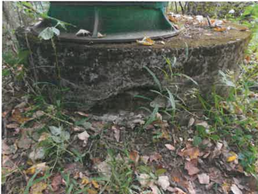
Manhole Identified for Replacement
