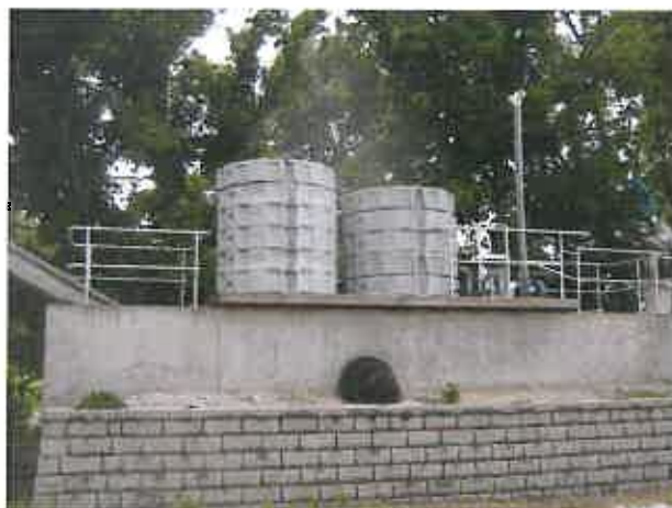
“Headworks” Facility with Scrubber Unit
