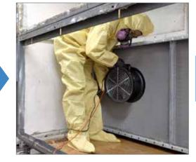
Pure Air Control Services Inc. performs their own proprietary Coil Cleanliness Verification Test (CCVT). This test is repeated across the span of the coils measuring the Delta P ( $\Delta$ P) to determine which zones of the coil are most fouled. This is helpful to report the before state of the coil, as well as letting the tech know which areas of the coil will require the most attention. The data is logged and then cleaning commences.
