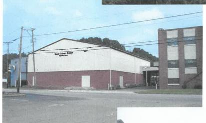
Structure is a pre-engineered metal building with a partial second floor and houses classrooms in addition to gym/multi-purpose room space.
