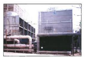
chilled water delivery system. Five roof-mounted induced draft cooling towers also have fans on variable frequency drives. The towers and building were configured for a final capacity of 8,000 tons.
