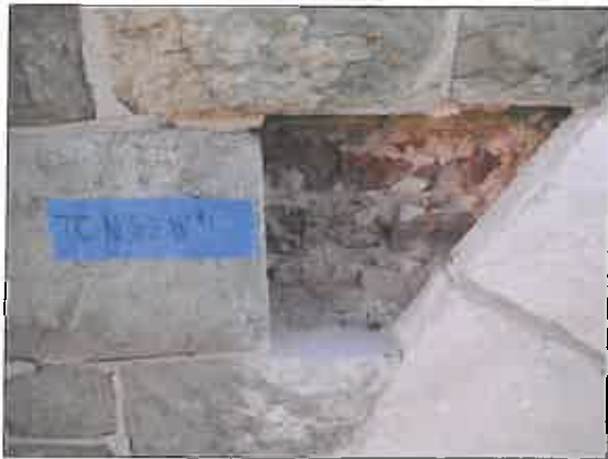
Exploratory opening within existing masonry wall assembly as part of field evaluation, St. Francis of Assisi
