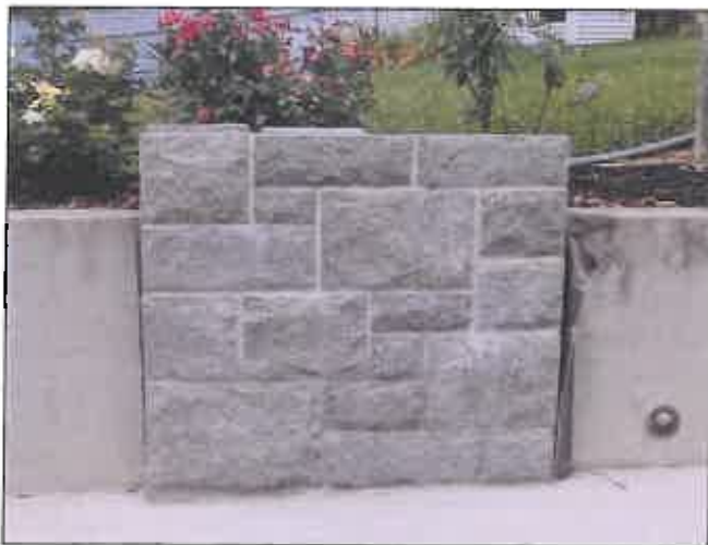
Reviewing a sample panel mockup with the VA SHPO for new stone façade for St. Francis of Assisi Catholic Church
