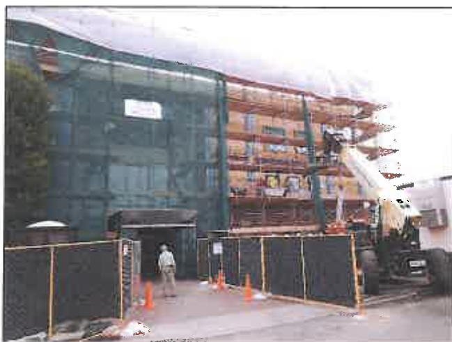
Overhead protection for building occupants at the entrance to the Public Service Commission Headquarters Building during construction
