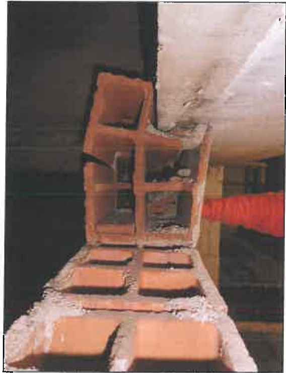
Investigation into Failures of Clay Tile Masonry – West Virginia State Capitol Building
