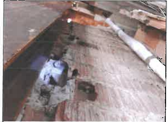
Evaluation of existing clay tile to develop shoring design Moynihan Train Station, New York City
